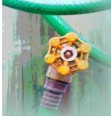
A cross connection is defined as an actual or potential connection between a public water supply and a source of possible contamination or pollution. All homes have potential cross connections.
